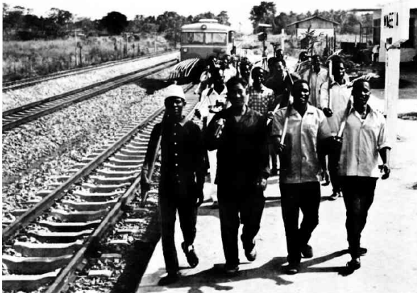
Tanzanian, Chinese, and Zambian workers set out to build the Tanzam Uhuru Railway. (Photo: Tanzanian Embassy)
